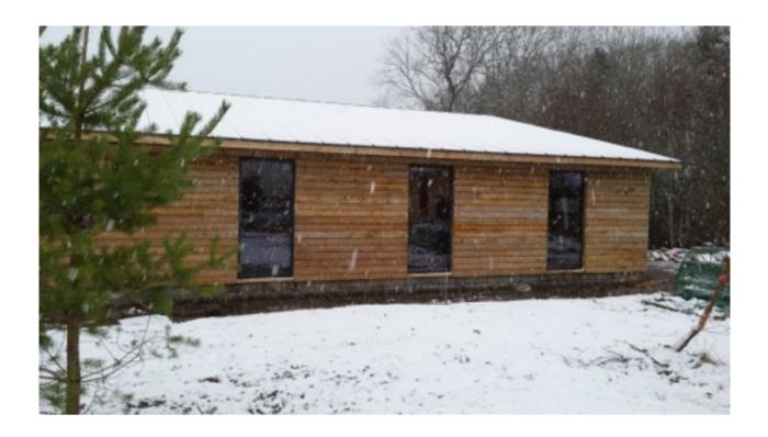
As the months went by the cladding began to weather, accelerated by the effect of the silica network forming in the surface substrate. This is a special attribute of the SiOO:X treatment.
