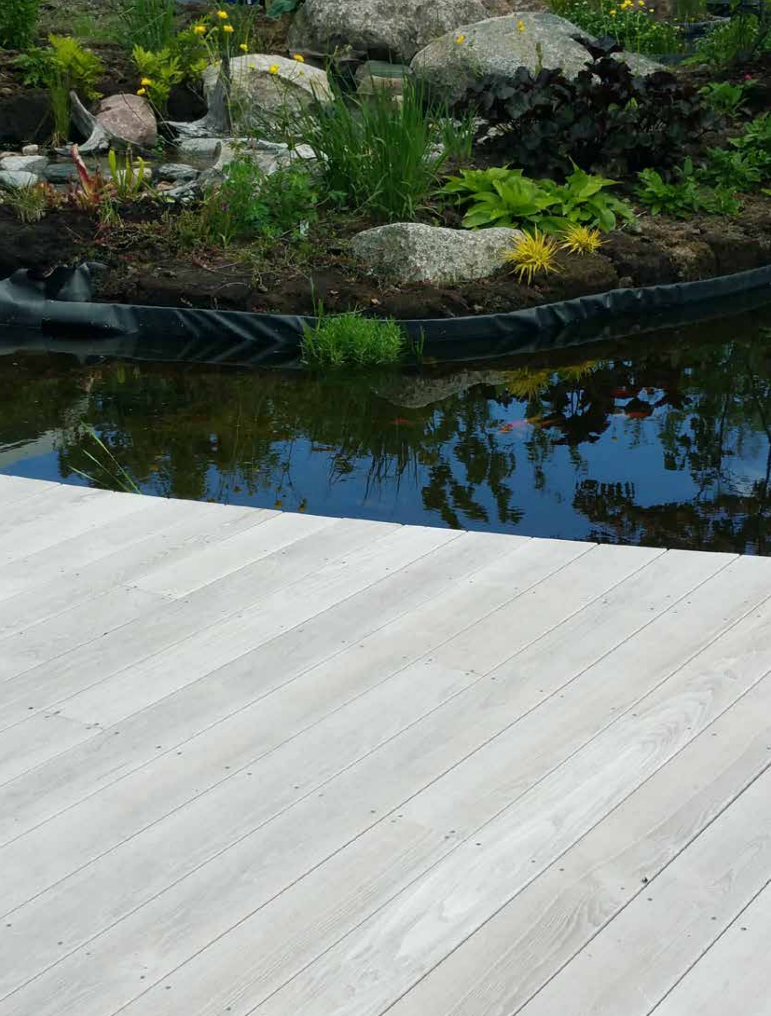
SiOO:X-treated deck, (in Svedala, Sweden) in Thermo Ash around 9 months after treatment. A similar appearance is obtained with Vulcan Decking.
